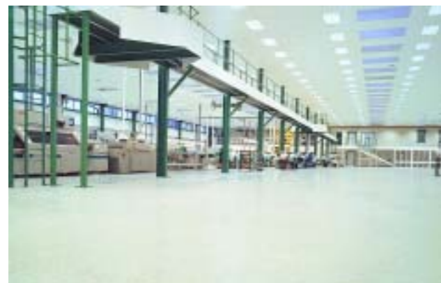
FINESSE EC - PRINTED CIRCUIT BOARD PRODUCTION FACILITY
