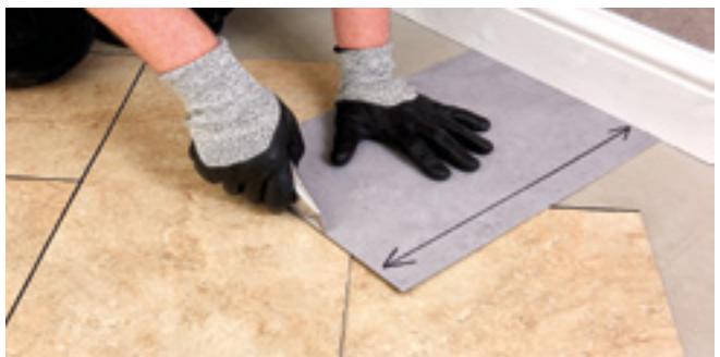
Figure 9 Cutting the perimeter tiles (diagonal cut)
