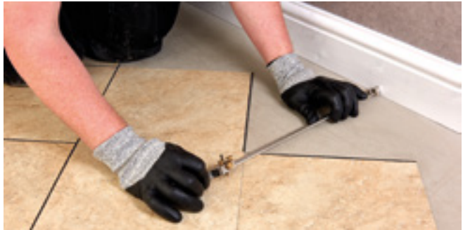
Figure 10 Cutting the tiles using a scriber (diagonal cut)
