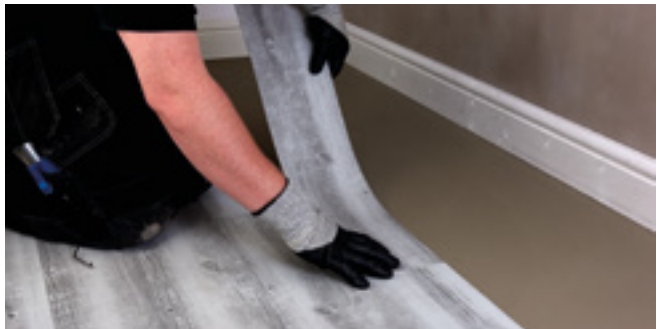
Figure 1 Setting planks out
